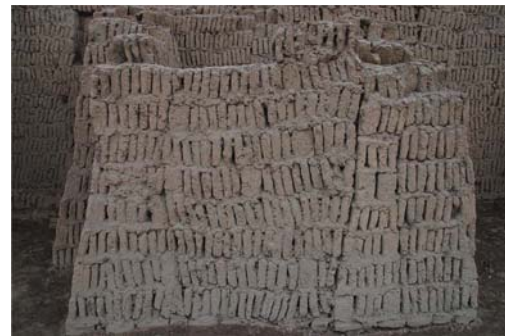
Figure 3. Detail of librillo bonds, with sloping walls profiles in Huaca Puccllana , archaeological site, Lima (Authors: Cristini & Ruiz Checa).
