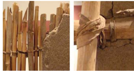
Figure 9. Detail of a quincha dividing wall, M. Antonini, Nazca (Authors: Cristini & Ruiz Checa).
