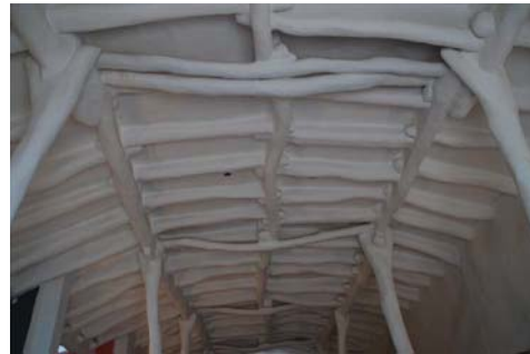
Figure 15. Example of contemporary house in Tucume, Chiclayo Province. A Guarango structure, with daubed earth and straw layers, lately whitewashed. (Cristini & Ruiz Checa).
