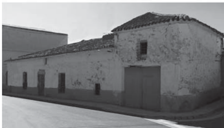
Figures 6 and 7. Case study in Navas de Jorquera (stone masonry wall) y Motilleja (rammed earth building) (Authors).
