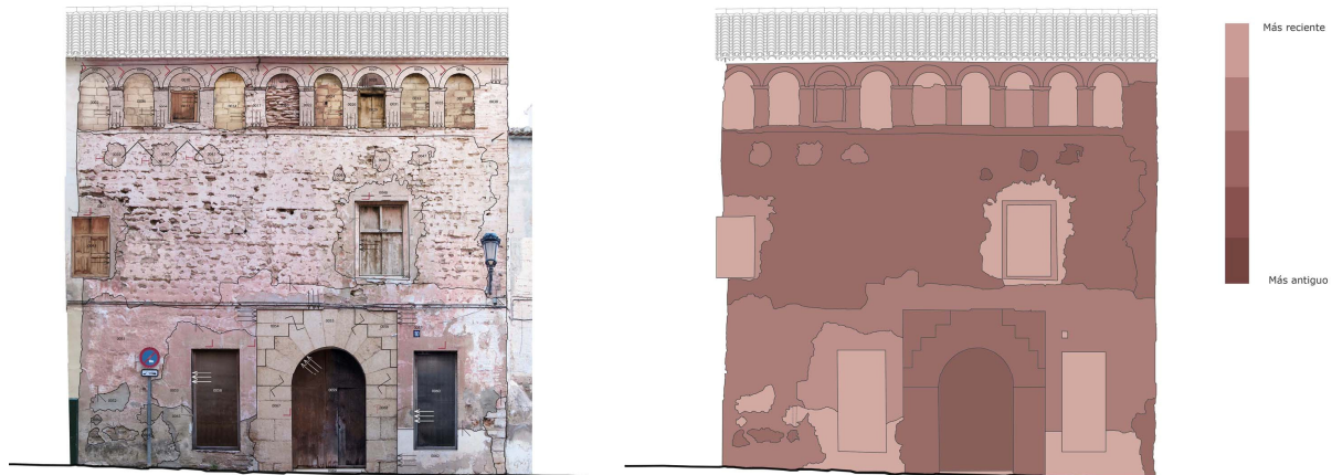
Fig. 3. Stratigraphical study of the building's façade. Practical work developed during the course 2010-2011 (Authors: M.A. de la Torre, B. Ferrer, A. García, A. Marí, I. Reig, M.J. Reig, R. Sola, C. Villalonga)
