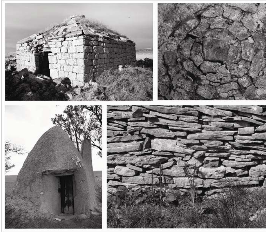
Figure 5 : Huts with corbelling domes built either with dry stone technique or plastered adobes
