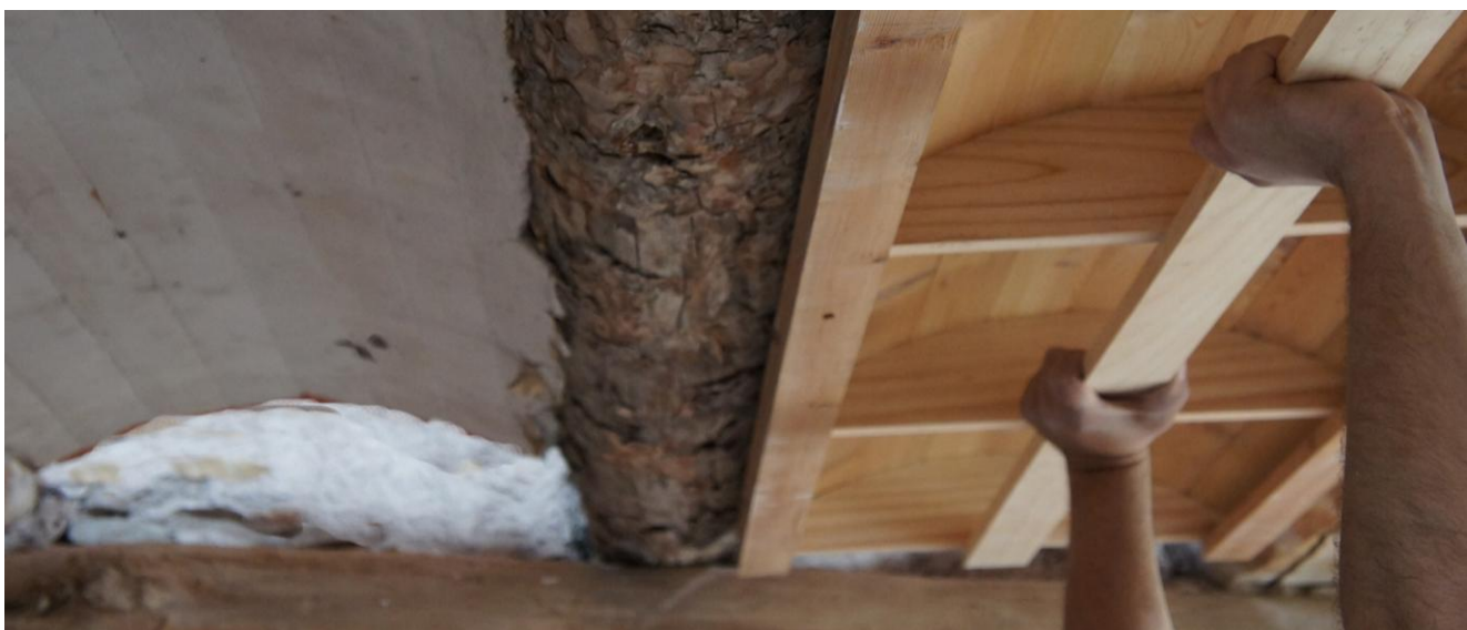
Figure 5. Reconstruction with new formwork for some missing vaults (Cristini)
