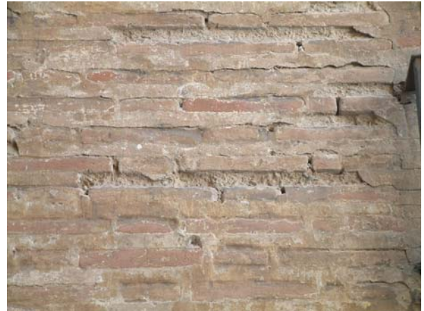
Figure 11. Detail of the facades' original treatment
