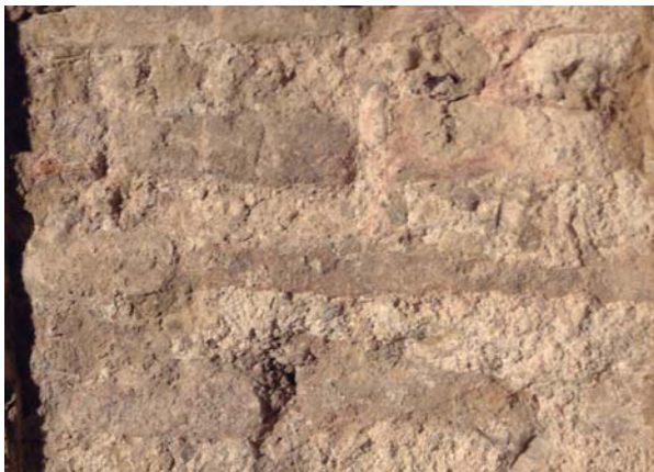
Figure 5. Detail of brick-reinforced pisé-de-terre techniques
