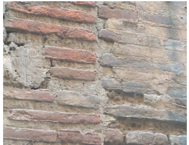
Figure 12. Imitation of the original treatment made during the intervention of 19 th century
