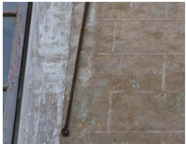
Figure 8. Detail of the treatment of false ashlars on the palace main facade
