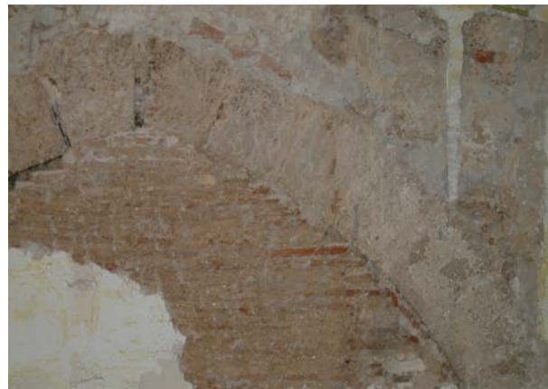
Figure 6. Ashlar arch subsequently filled with brick fabric
