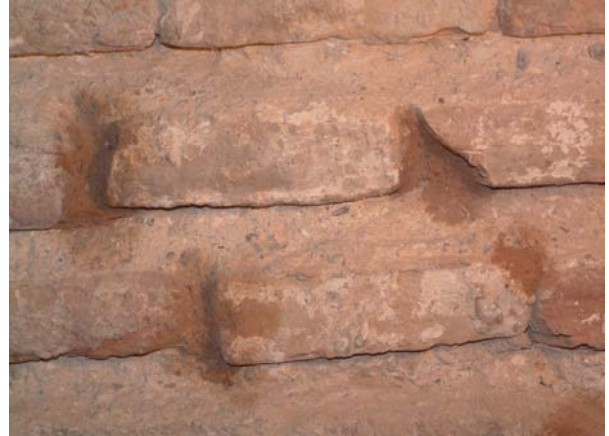
Figure 13. Selective rejoining made only in the vertical joints
