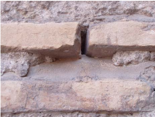
Figure 2. Communion Chapel of the Church de Santos Juanes (1644). Detail of agramilado method that shows the first layer of the joint and rests of the sealing second layer called zaboyado .
