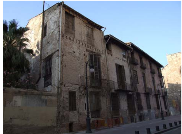
Figure 7. Rear facade of the Calle Exarchs palaces
