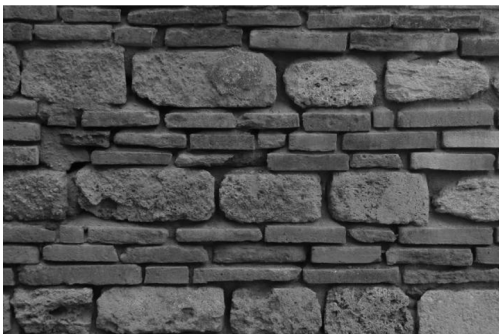
Figure 10. Opus mixtum with alternating layers of bricks and stones, Istanbul, Turkey (Cristini).
