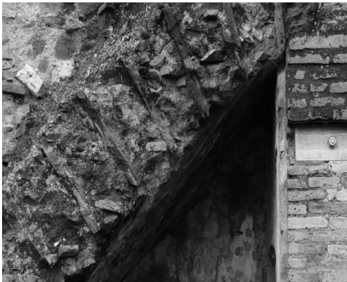
Figure 9. Bricks connectors, Livia's House, Rome, Italy (Cristini).
