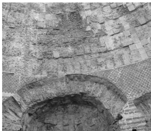
Figures 7–8. Brick linings on the intrados of vaults prevented wooden frames from adhering to the concrete after it had cured Villa Adriana, Italy (Cristini).
