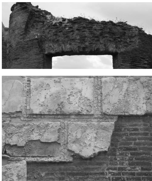
Figures 1–2. Details about opus testaceum and fake stones treatment, Pompei, Italy (Cristini-Ruiz).
