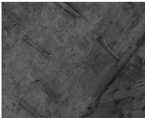
Figure 6. Bricks on the intrados of vaults, thermae of Villa Adriana, Italy (Ruiz).
