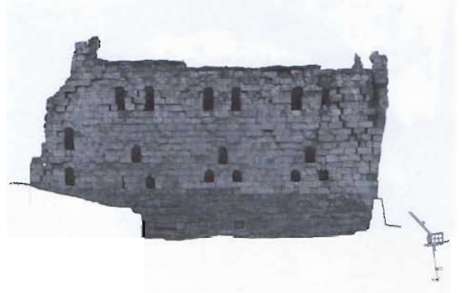
Figure 7 Metric lifting. Example of the photographic rectification. Detail of the east face.
