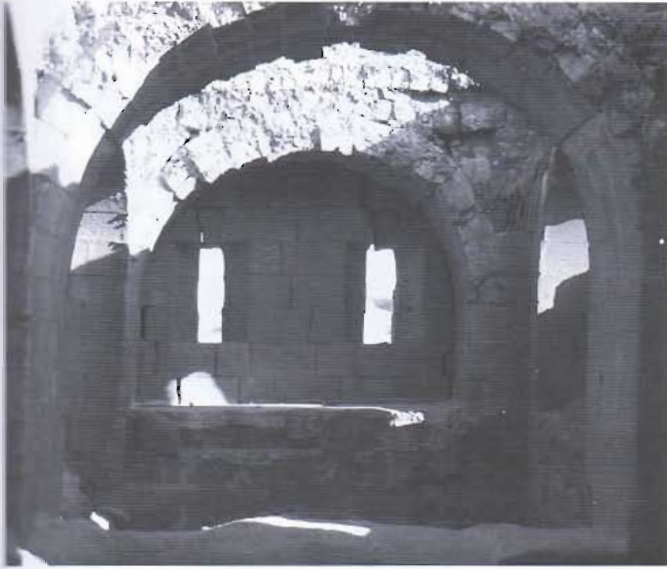
Figure 3 Details inside the gallery.
