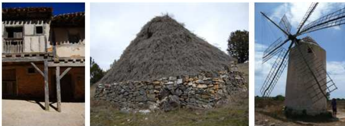
Fig.1 (from the left) Examples of juniper timber in vernacular architecture: pillars, thatched roof, mil (RUIZ CRISTINI)
