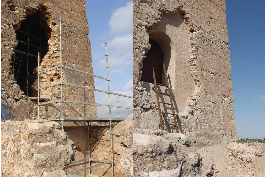
Figure 7. Reintegration works respecting the detail without having an impact on the overall view of the building (Cristini).
