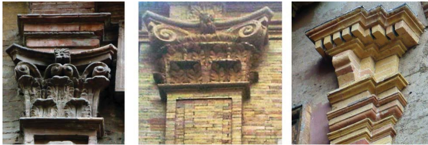
Fig.4 Scrolled volutes and capitals with “marly” bricks: Condes de Alpuentes Palace, Communion Chapel in St Martin Church, Royal Basilica, Valencia (Cristini; Ruiz-Checa)
