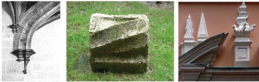
Fig.1 From stone virtuositities to brick technical details. Gothic details from La Trinidad and Santo Domingo Monasteries (Gotichmed [4]) and Marques de Campo façade (Cristini; Ruiz-Checa)
