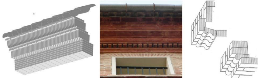
Fig.3 Cornices and dentils: Pineda Palace details and common solutions visible in Valencia City Centre (Cristini; Ruiz-Checa)
